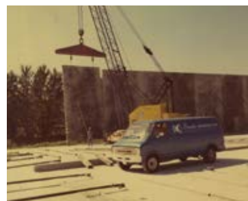
Innovative tilt-up industrial construction method / 1960s
